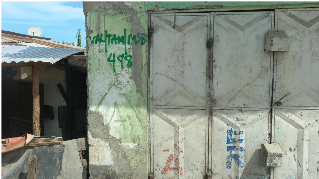
Figure 7-1: Example of marked structure
